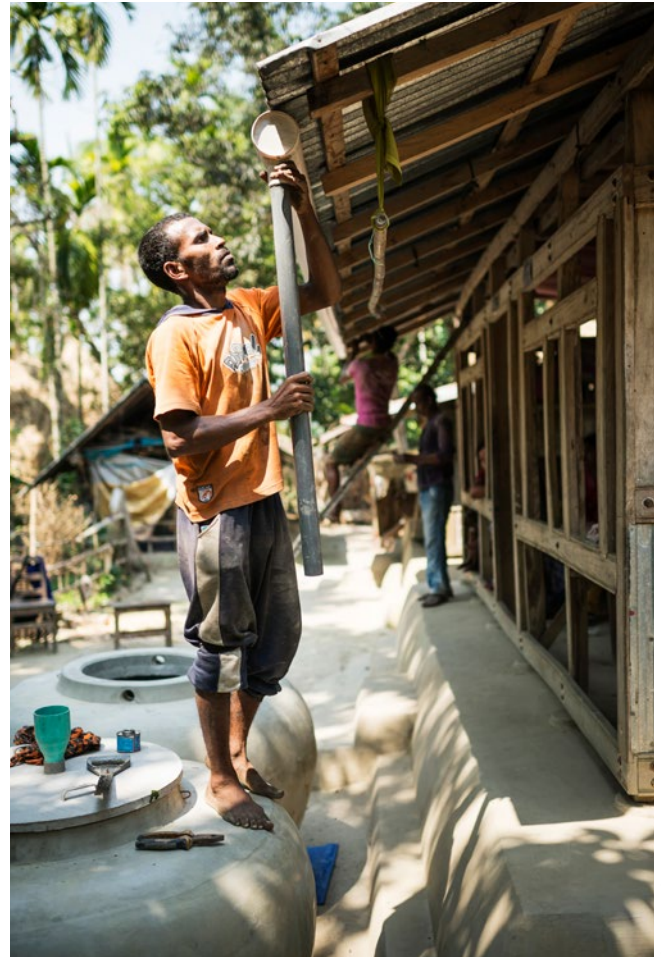
Installation of rainwater harvesting system in Bangladesh
