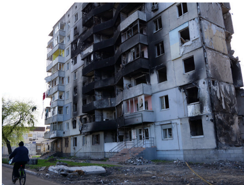
Destroyed residential buildings in East – Ukraine after an attack through the Russian army. Photo: Alyona Budagovska
