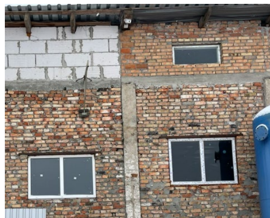
Industrial Building in Makariv, made of reused bricks
