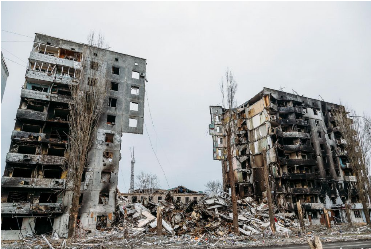
Collapsed Khrushchevka Building in Borodyanka
