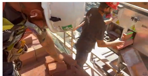
In-Situ brick trimming in Canada Image: Youtube
