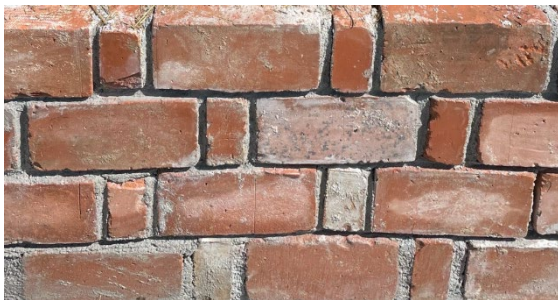
Rowlock Bond with reclaimed bricks and waste-based insulation (Balkans, SDC, HEKS, VoRAE, Skat) I: D. Wyss
