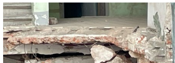
An old slab in Kharkiv, made of concrete and old bricks
