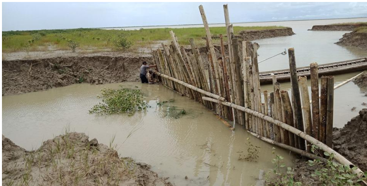
The local conservation group built a fence to protect the mangrove area from the sea tide.
