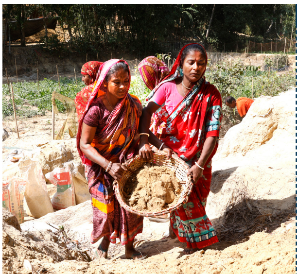
Community road rehabilitation ©Helvetas/Franca Roiatti
