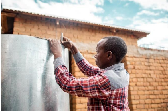
Faraji Mwahu, artisan from Bolisa ward Kondoa district preparing the base of a metal silo before fixing the cover
