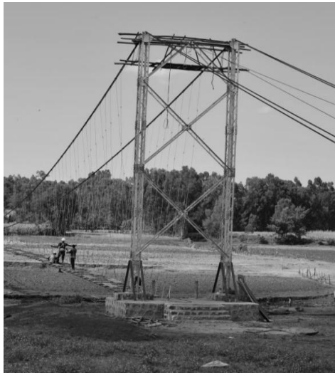
Figure 5. Steel tower, Rwanda style
