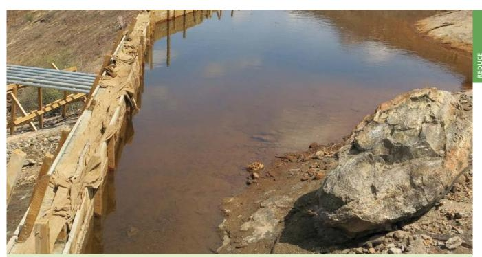
Community rock catchment under construction in Ndikir village, Marsabit County, Kenya. The weir dams hold surface runoff when it rains, channeling the water into a piping system which leads the water into masonry storage tanks (Fredrick Ochieng).
